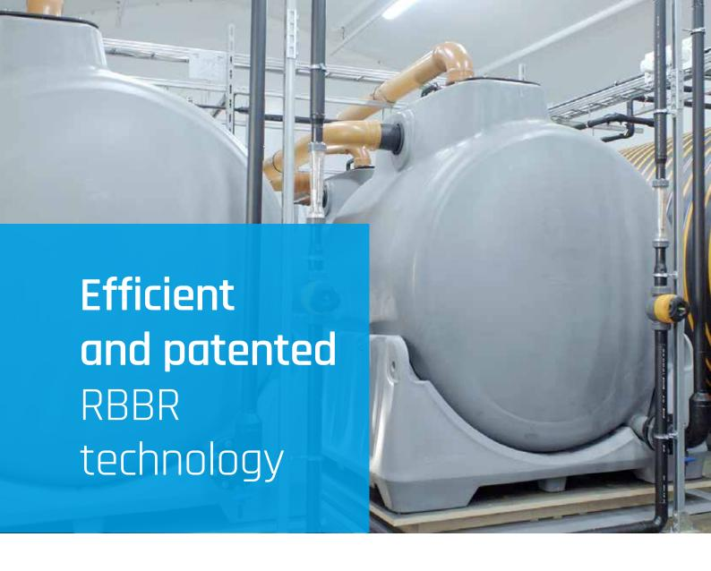
Clewer's waste water treatment systems use a Rotating Bed Biofilm Reactor (RBBR), a patented next-generation biofilm reactor developed in Finland.
